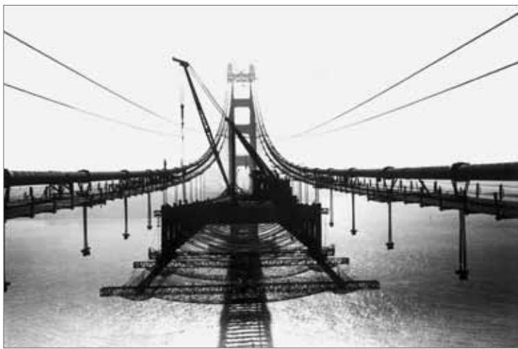
Golden Gate Bridge im Bau, Sicherheitsnetze, 1936, Foto: From the holdings of the Golden Gate Bridge, Highway and Transportation District, used with permission, www.goldengate.org
